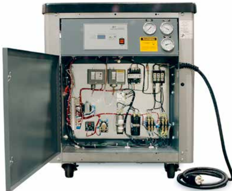
Typical Electrical Panel : 2 ton units
