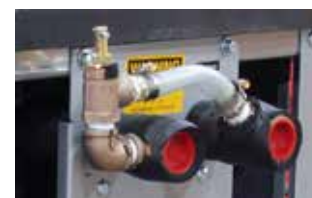
Typical automatic low flow bypass valve.
