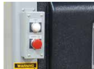
Emergency stop button. Shown with Power On light.
