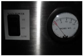
Through use, a slow steady deflection to the right will occur; this indicates the prefilter filter is working. As the gauge approaches 2.0 in of water column the pre-filter filter needs to be changed.
