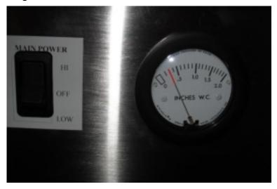
This is a differential pressure gauge. From this point of calibration, a 100% blockage of the filters will yield a reading of .5 in of W.C. At that time the pre filters and other filter media should be changed.
